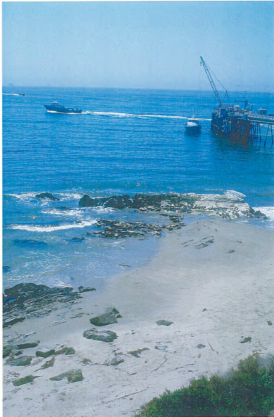
FIG. V-4. SANTA BARBARA CO., CARPINTERIA. At Chevron Point, Carpinteria, the marine system is a valuable component of petroleum-based activities. The pier (upper right) is an intermediate between the offshore oil platforms and onshore refineries. Also shown (center) is the function of ocean beaches as haul-out and pupping grounds for harbor seals ( Phoca vitulina ), despite their proximity to the noise and activities associated with the boats and pier. (See also Fig. V-12).
