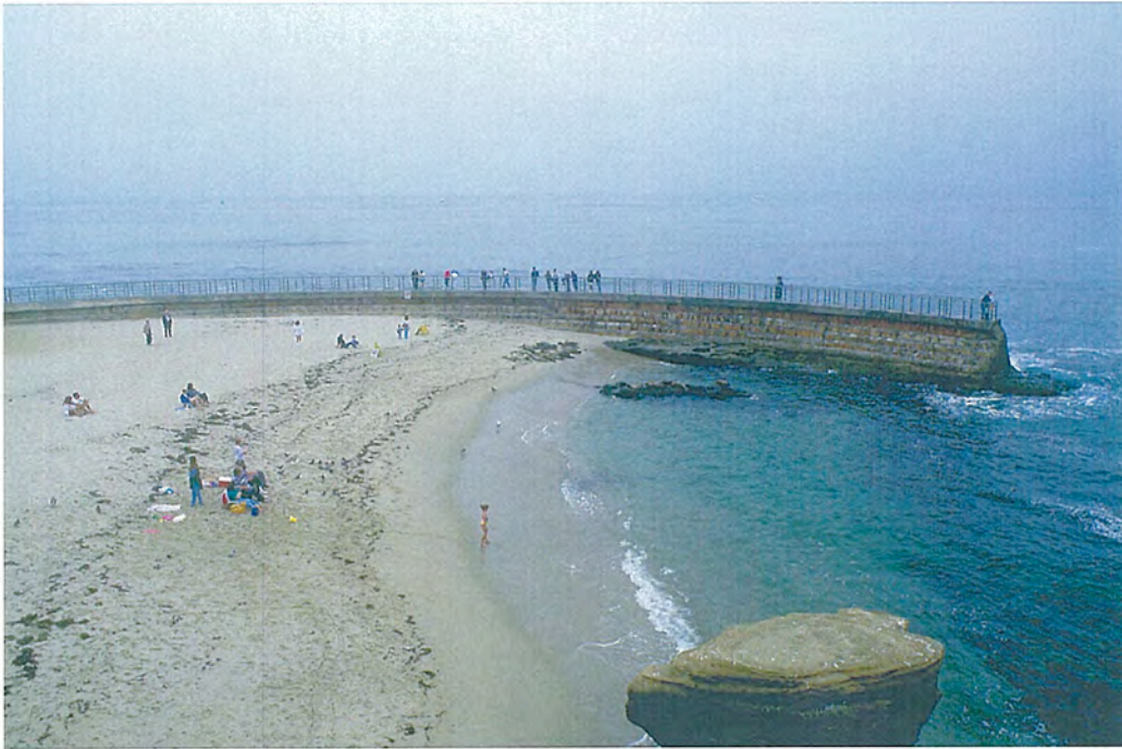
FIG. V-30. MARINE-INTERTIDAL UNCONSOLIDATED-SHORE (SAND) REGULARLY-FLOODED COVE-BEACH WETLAND. San Diego Co., La Jolla, along Coast Blvd., Children's Pool. When the seawall was built, the longshore current filled this artificial cove with sand, creating a protected beach on an otherwise exposed and cliff-faced coast along La Jolla bluffs.
